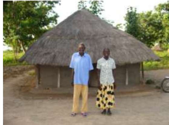
CCMP members at their old leaking but in lire parish.
