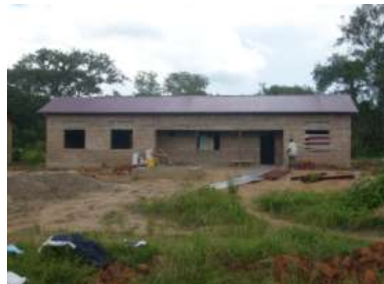
An Office block under construction in Sodogo.
