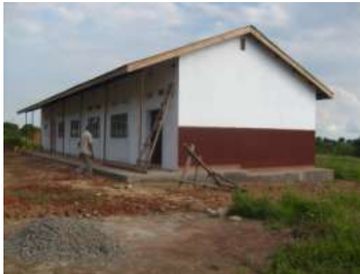
The New College Kitchen/Dinning Hall under construction – just about finished.
